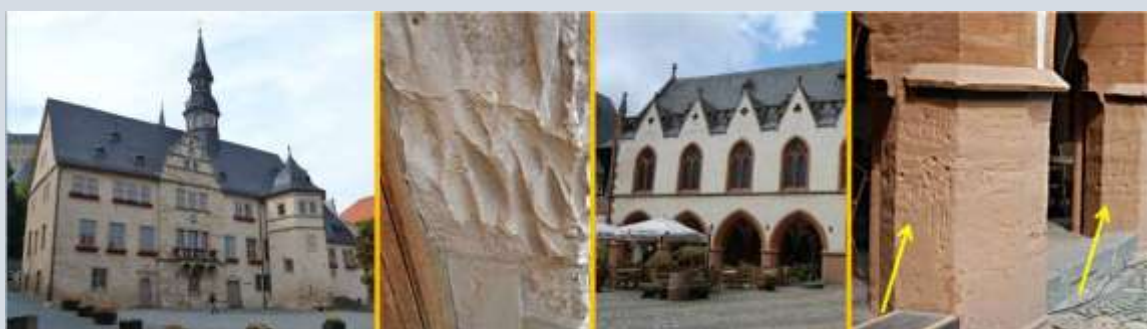
Scratch marks in the town halls of Blankenburg (photo 1+2) and Goslar (photo 3+4), both in Germany
