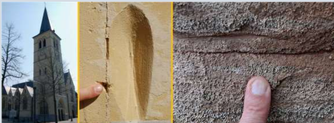
Scratch marks in limestone ('marl') in Bree in Belgium (photo 1+2) and in Rogenstein in Braunschweig in Germany (photo 3)
