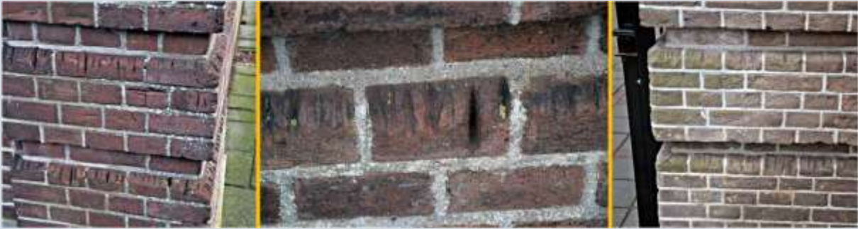
A phenomenon that resembles scratch marks: grinding grooves created by pencils for writing on slate.
