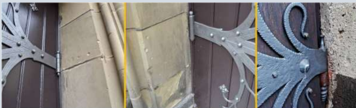
A phenomenon that resembles scratch marks: pseudo cups that are formed by the round heads of bolts that attach the hinges of doors.
